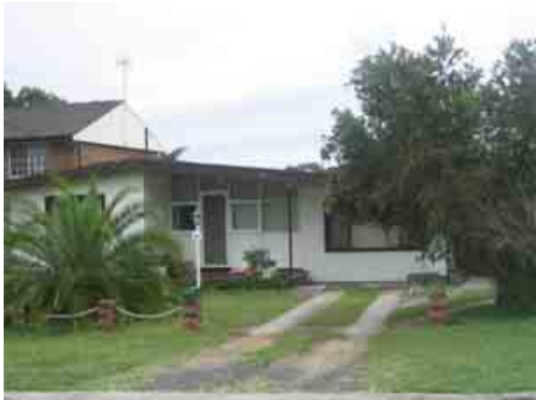
Fig 5.15.1 Existing residential dwelling at Liddel Street (Source: Dickson Rothschild)
