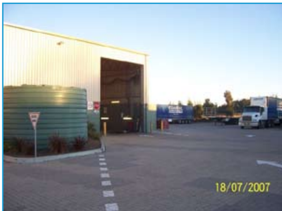
Truck wash facility
