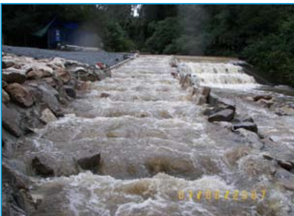
Upper Ourimbah Creek fishway
