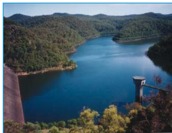
Mangrove Creek Dam
