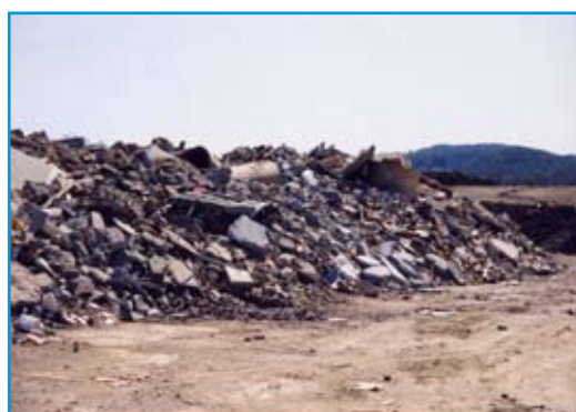
Bulk concrete recycling
