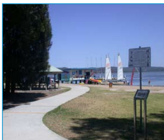
Some of the off-road cycleway which has been constructed at North Entrance
