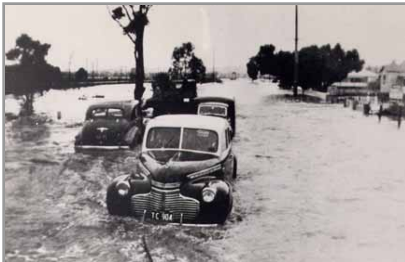
Figure 5: Historical flooding in Tuggerah Straight (1949). The Pacific Highway looking south (photo courtesy of David Williams).
