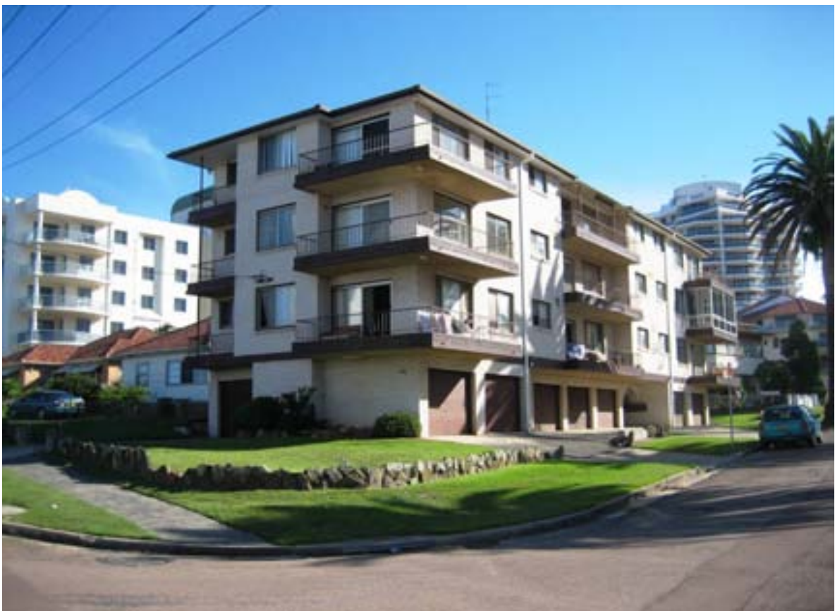
Neighbouring units at the corner of Bayview Avenue and Ocean Parade
