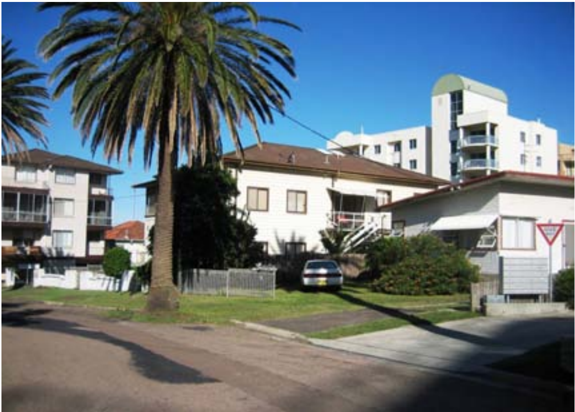
Bayview Avenue frontage
