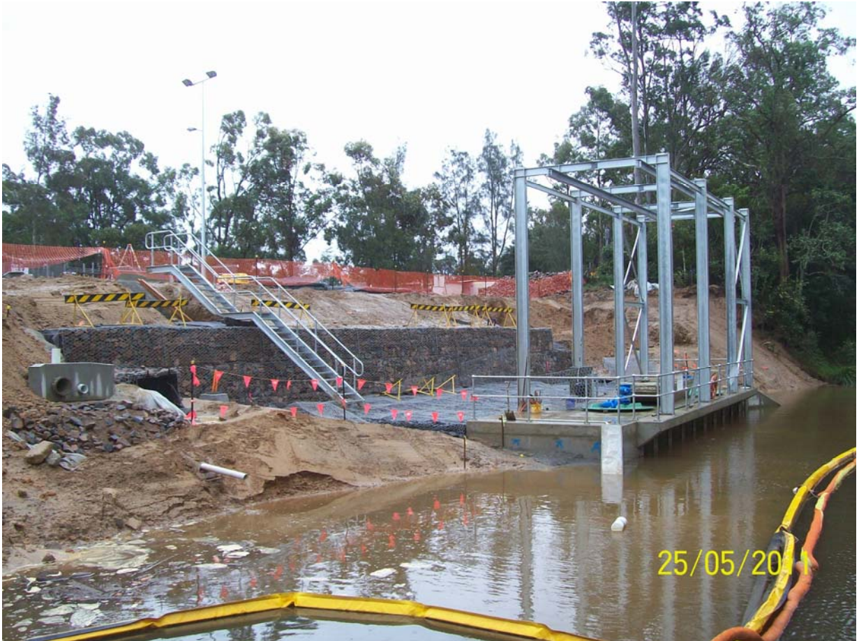
Wyong River Off-take Structure nearing completion (Work Package 1)
