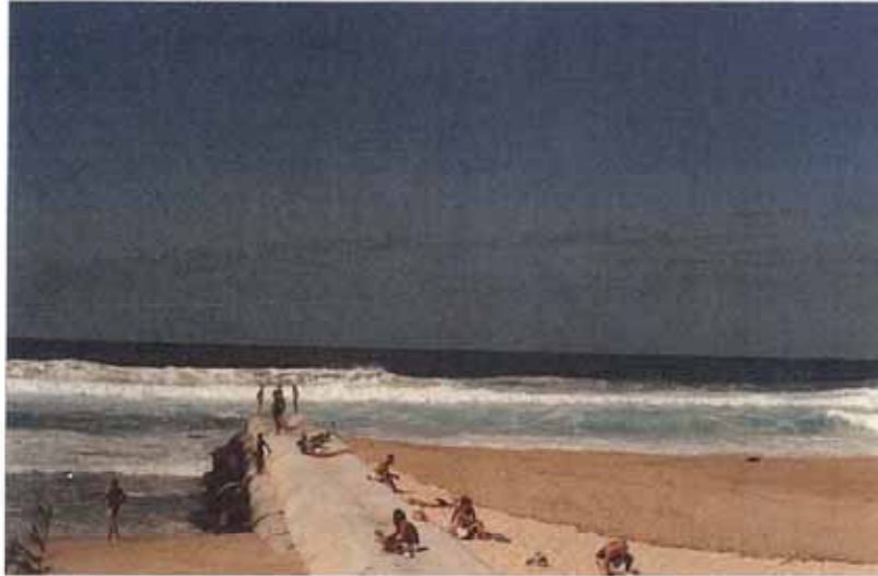
Fig. 1. North Kirra Groyne
