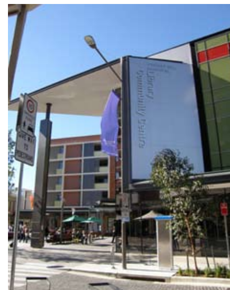
Above: Gateway building with active uses on ground floor. Below: Community building/library with plaza forecourt.
