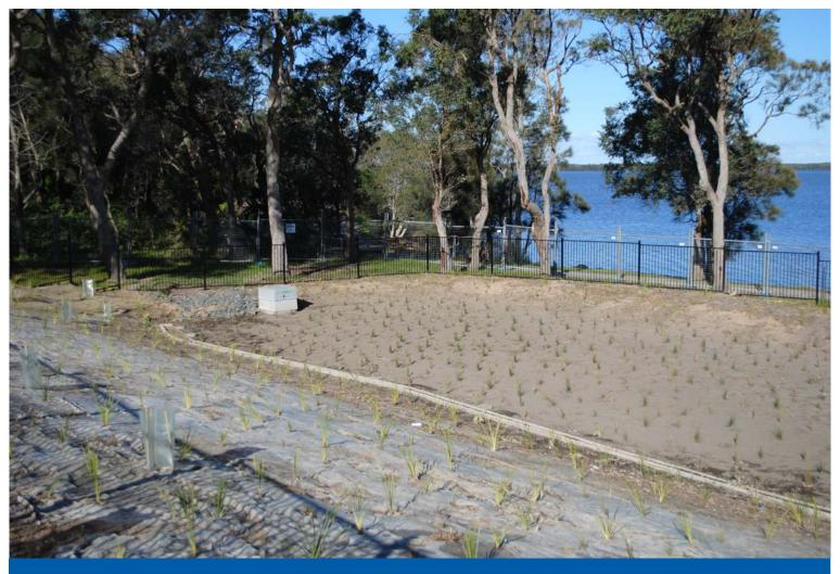
Construction of a rain garden and Gross Pollutant Trap to filter stormwater before it flows in to Lake Munmorah is almost complete. The works are part of the Tuggerah Lakes Estuary Management Plan.
