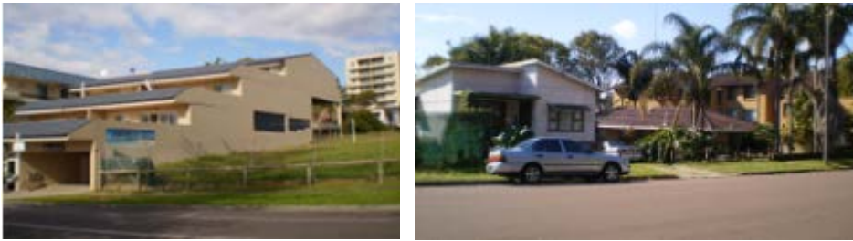
Above: Photo of eastern boundary from Marine Parade (left) and from Ocean Parade (right)
