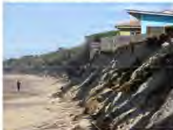
Figure 3.1. Erosion at Old Bar, Taree (7 July 2008).
