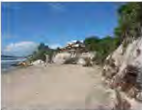
Figure 2.1. Erosion at Belongil Spit, Byron Bay (2 June 2009).
