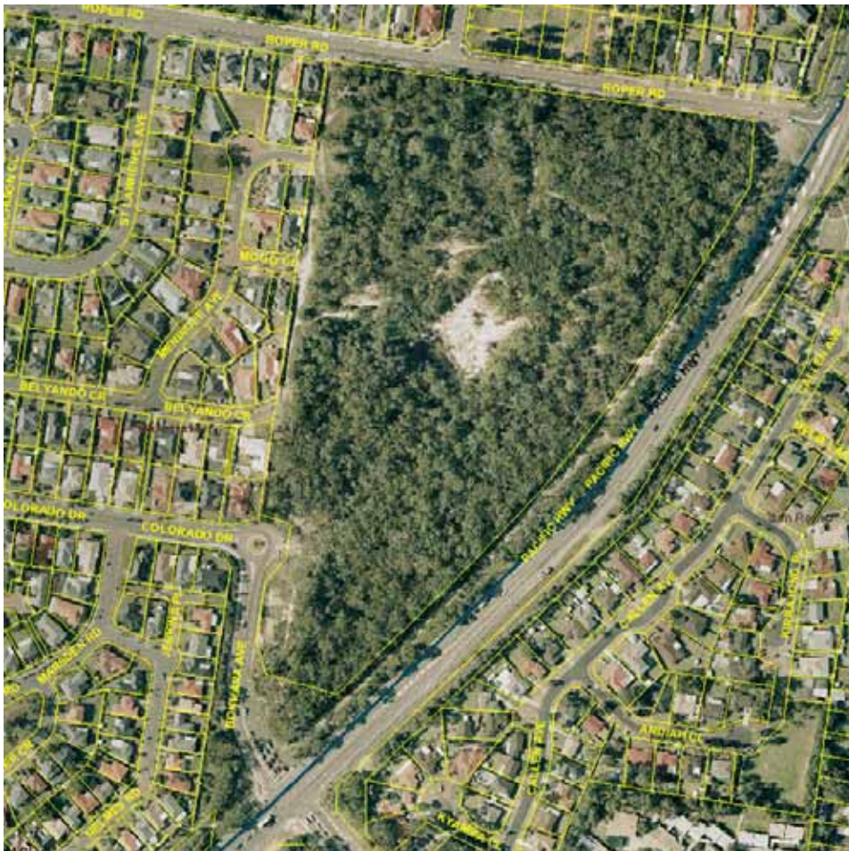
Aerial view of site – Blue Haven estate to left and Pacific Highway to right of view
