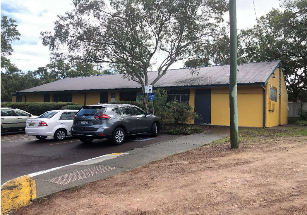
Figure 2 – View of building to be extended
