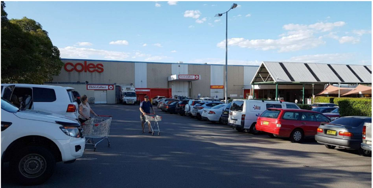
Figure 11 – Existing Coles southern elevation
