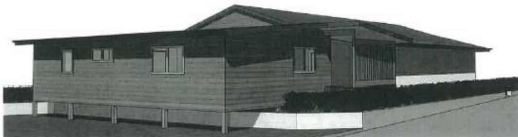
Figure 4 – External view (of north-western end)
