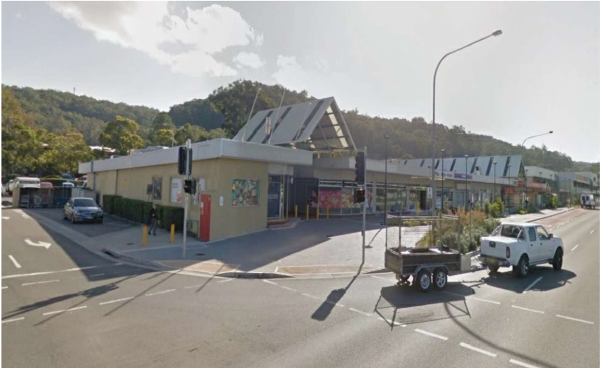
Figure 13 – Existing south eastern elevation at the intersection of Brisbane Water Drive
