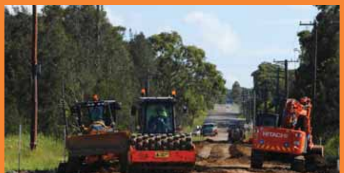
Minnesota Road Upgrade
