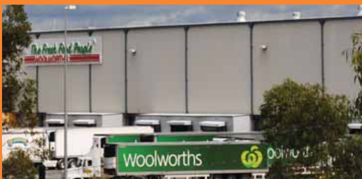
Woolworths Distribution Centre
