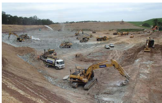
Construction of new waste cell at Buttonderry Landfill
