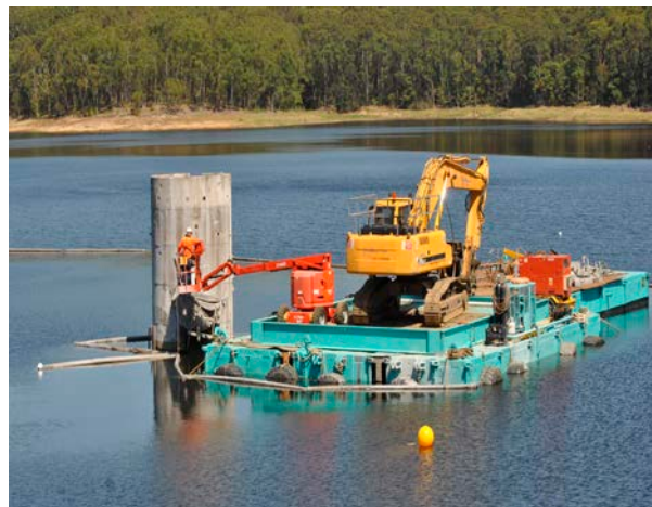
Demolition work at Mardi Dam
