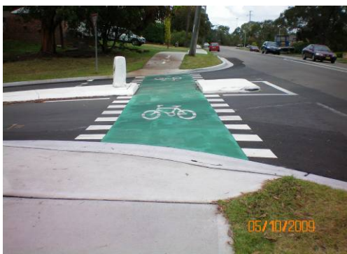
Figure 3.5 - Road crossing containing rolled kerbs, surface paint and line marking treatment linking two shared pathways
