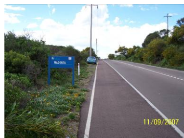
Figure 3.2b: Quality surface on-road bicycle lane
