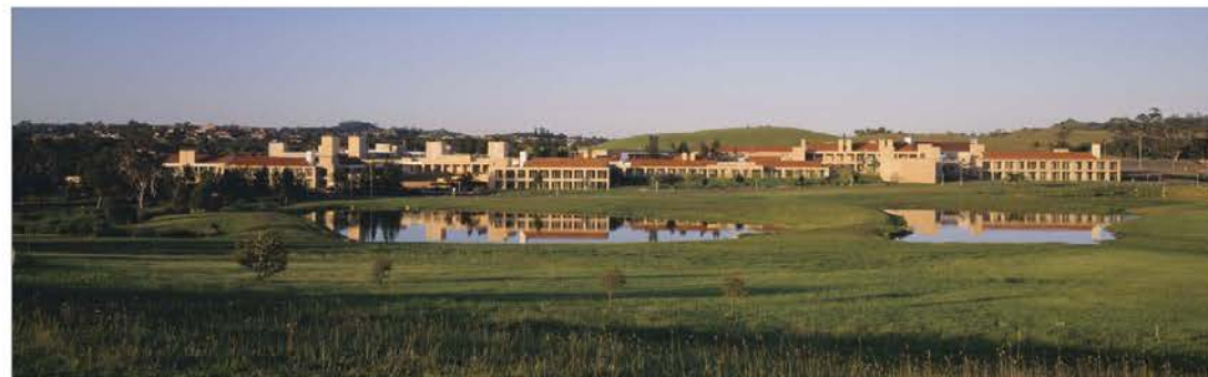
Figure 26 - University of Western Sydney - Campbelltown, Macarthur Campus - another greenfield university campus of a similar size and scale.
