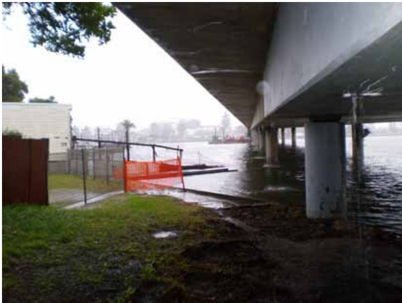
View from under The Entrance Bridge looking south toward the subject site and reclaimed Crown Land
