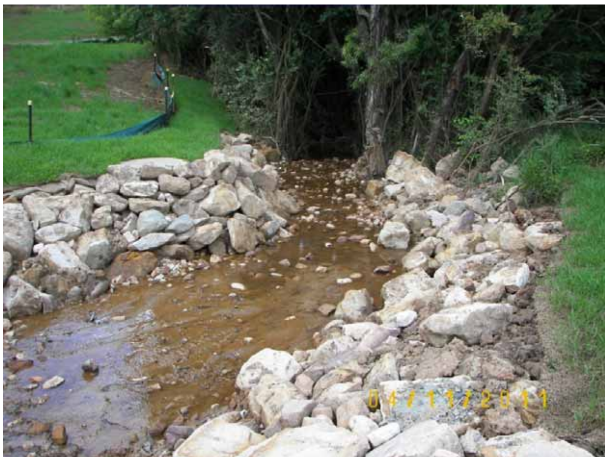
WP 07 restoration of creek crossing (Work Package 7)
