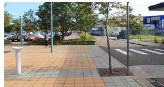
Existing concrete unit pavement - Main Street and Village Green
