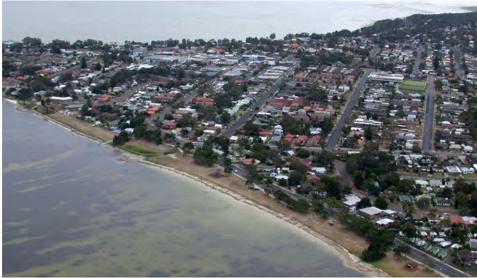
Photo 11: Aerial view looking north across Toukley
