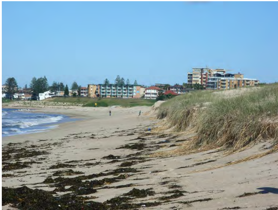
Photo 13: Storm damage, North Entrance
