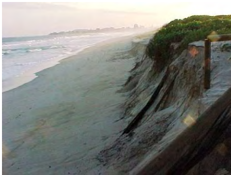
Photo 18: Coastal storm damage
