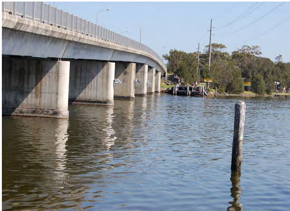
Photo 12: Toukley Bridge looking west
