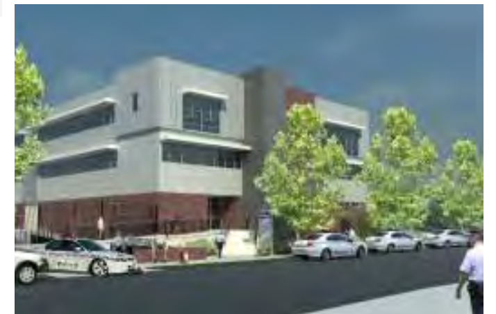
Regional Police Station (Under Construction)
