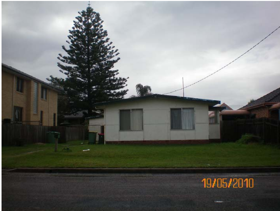
Figure 2: Property frontage showing existing dwelling to be demolished.
