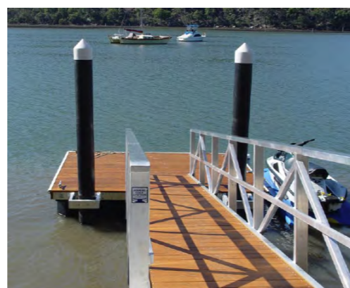
Floating timber pontoon example
