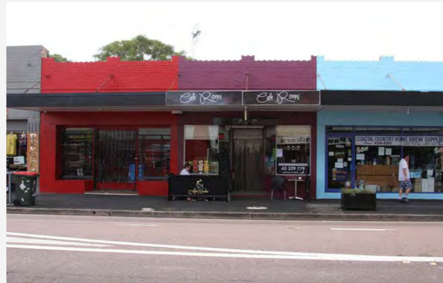
Building Facade Painting along The Entrance Road
