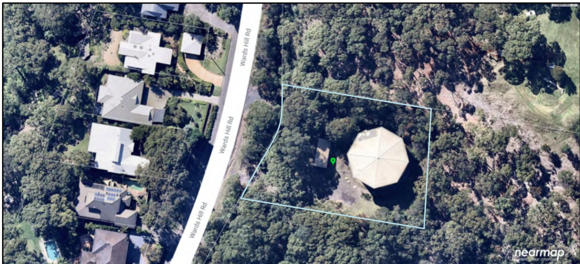
Figure 2: Aerial Photograph of Subject Site (outlined in blue) – Source Nearmap
