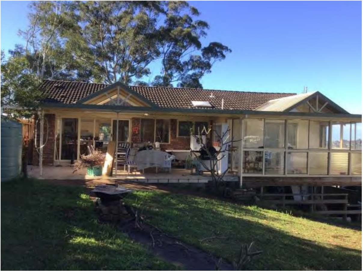
Figure 4 – Photograph of existing rear façade.
