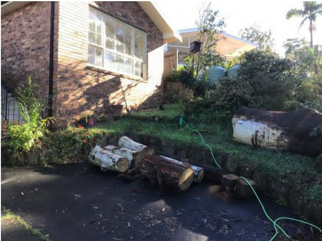
Figure 3 – Photograph of existing front façade looking more northwards where carport is proposed.
