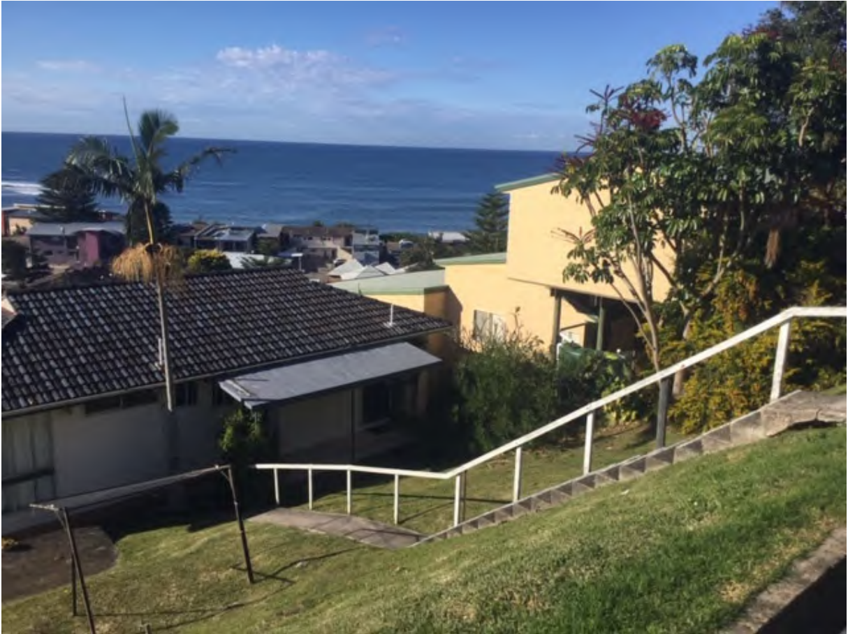
Figure 4: Photo taken from road of existing white weatherboard clad and blue/grey tiled roof to be demolished
