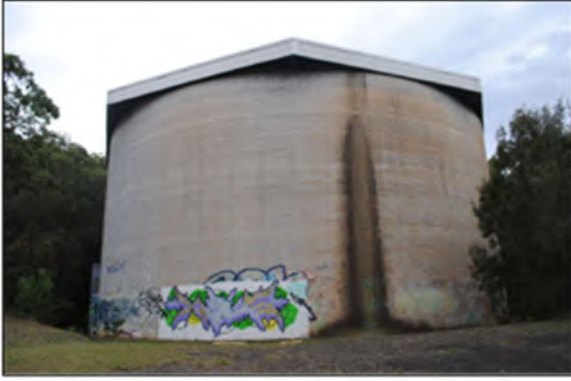
Figure 5: Photograph of existing reservoir tank
