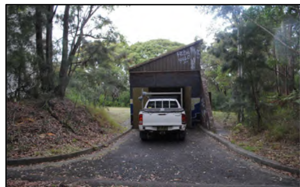
Figure 4: Photograph of existing electrical building looking south
