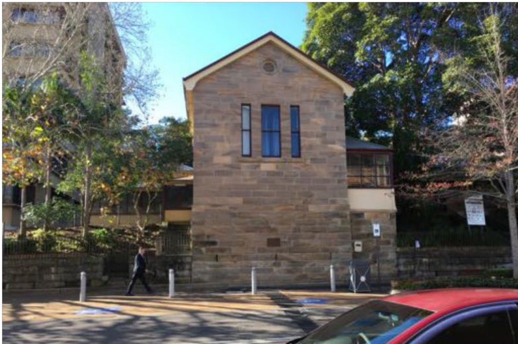
Figure 5: Subject Site: Exterior of Robert Knox Hall viewed from Mann St.
