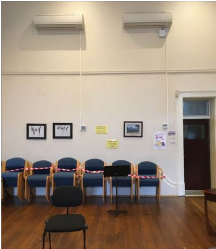
Figure 13: Subject Site: Existing Robert Knox Hall, Eastern internal face.
