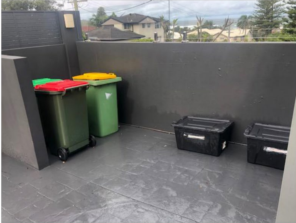
Photograph 3: Existing Waste Store.
