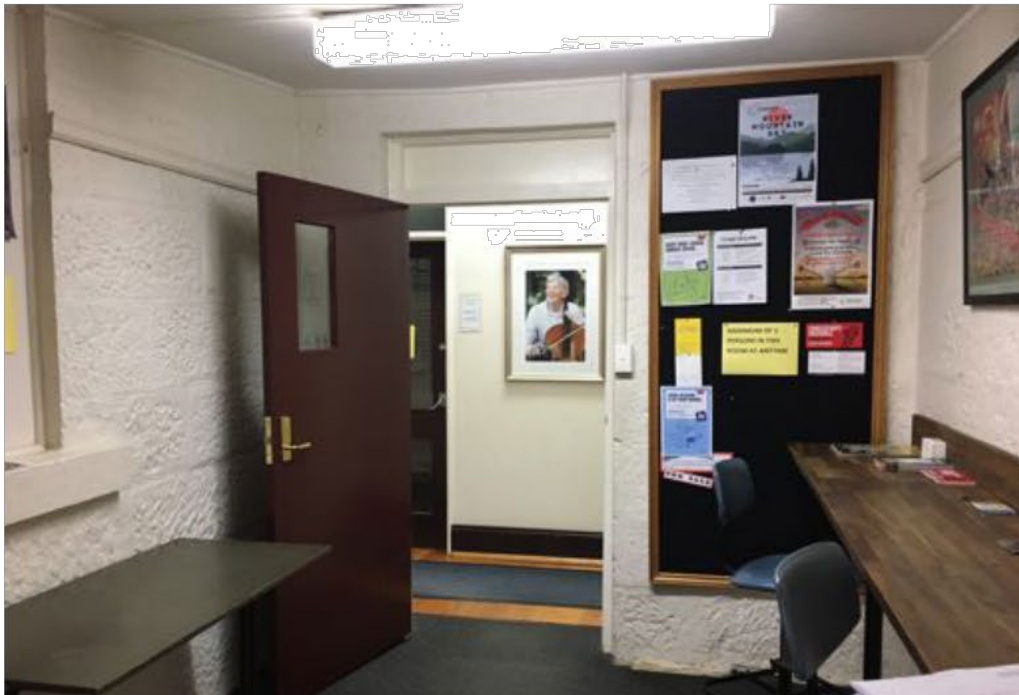
Figure 10: Subject Site: Internal rear access to be opened to provide new foyer connecting Mann street and Georgina terrace.
