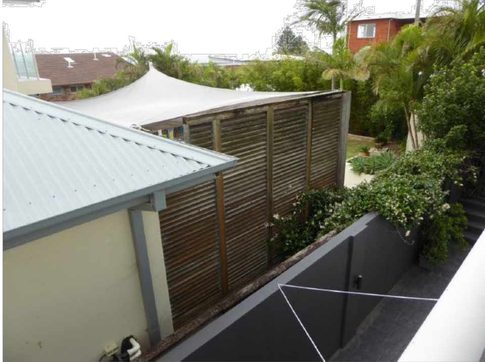
Photo 9: Privacy Screen – No. 10 Dover Road.
