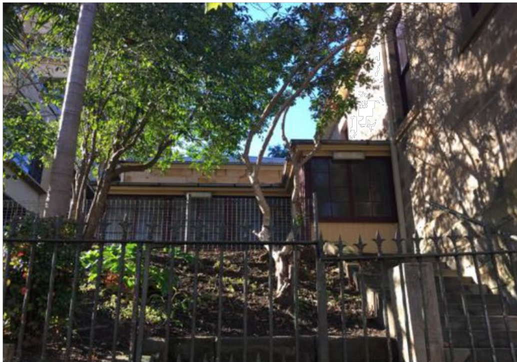
Figure 3: Subject Site – Mann Street addition to be upgraded.
