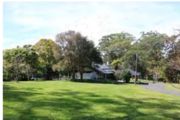
G. VIEW OF HOMESTEAD LOOKING NORTH EAST
