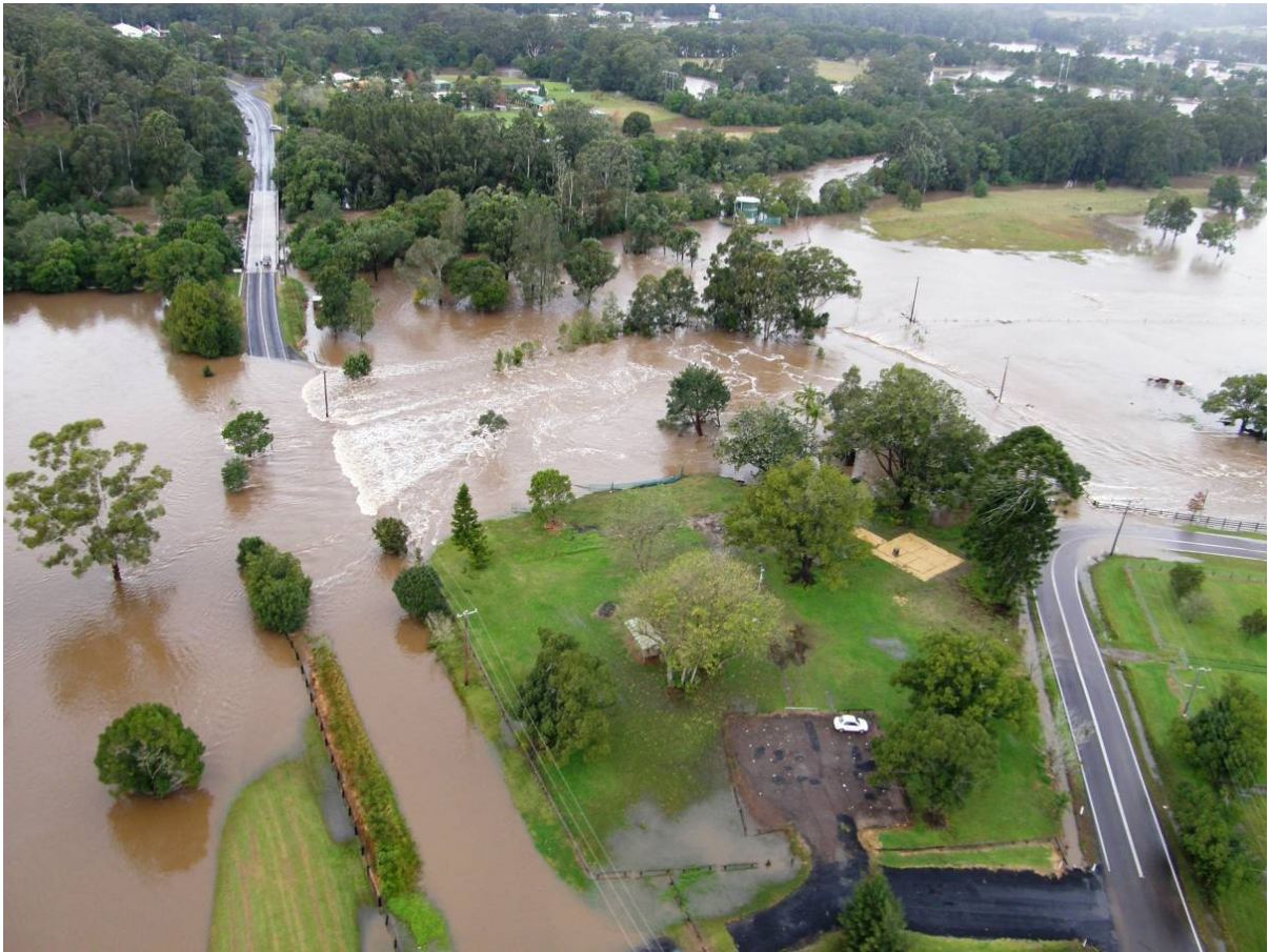
FIGURE 4 –Observing Alison Road river crossing approximately 1.5km west of the development, looking eastward, on 9 June 2007. The predicted 1% AEP flood level is 2.6m higher than the water level pictured.
