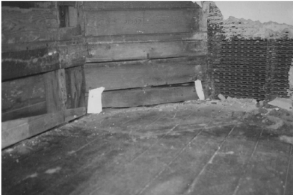
Plate 6: The Homestead in the 1980's noting the remnant timber lining boards adjacent to the lath and plaster walls. (Source - WDM&HS)
