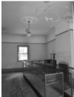
Plate 14: Room 1 showing signs of damage to the ceiling and the fire mantle and box removed.
