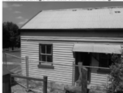
Plate 26: Salvage weatherboards for re-use.
