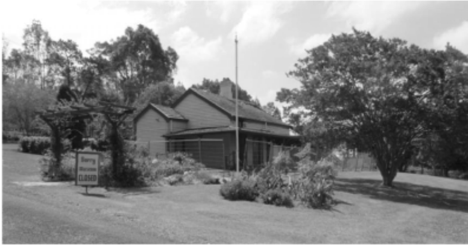
Plate 31: The proposed pavilion to be retained as part of the redevelopment of the site.
