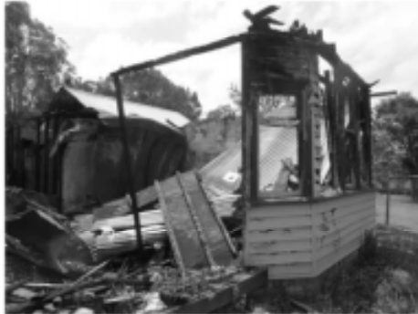
Plate 19: The remains of the bay window to Room 6.
