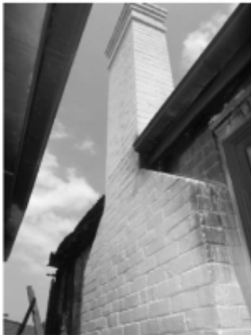
Plate 23: Chimney to Rooms 8 & 9.
