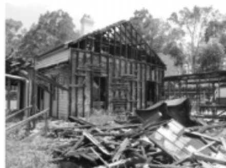
Plate 18: View back to Room 2. Note; hardwood weatherboards slowed the fire damage
