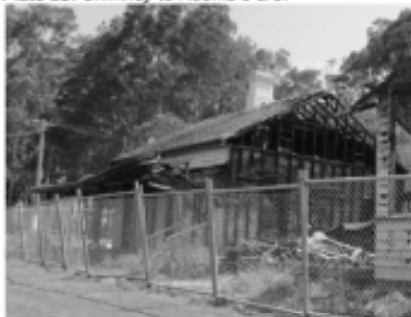
Plate 25: Salvage tiles from roof for re-use.
