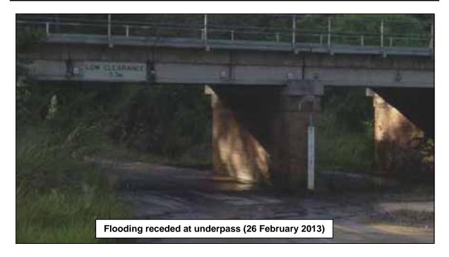
From recorded rainfall data it is estimated that the 2.0m flood depth observed on 29 January 2013 at the underpass was about a 50% AEP (1 in 2y) flood event, as shown below:
