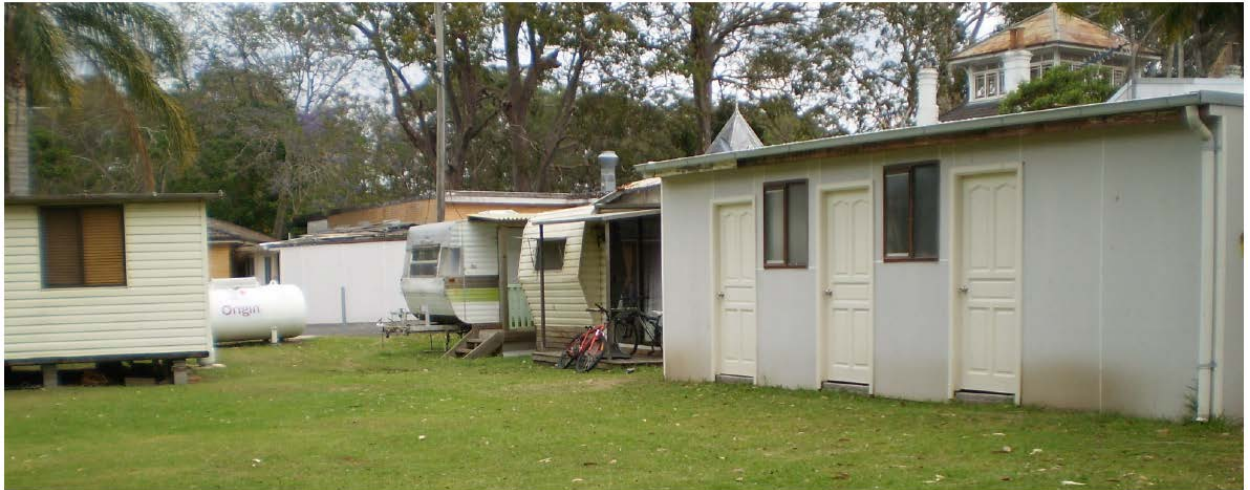
Above: Mobile home (left), two caravans and annexes (8 and 9), unauthorised conversion of shed to boarding house accommodation (right) and turret of Strathavon lodge (background).
