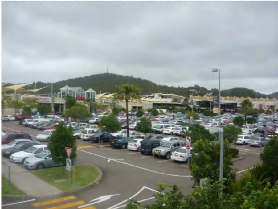
Figure 6. Westfield shopping centre and parking area at Tuggerah
