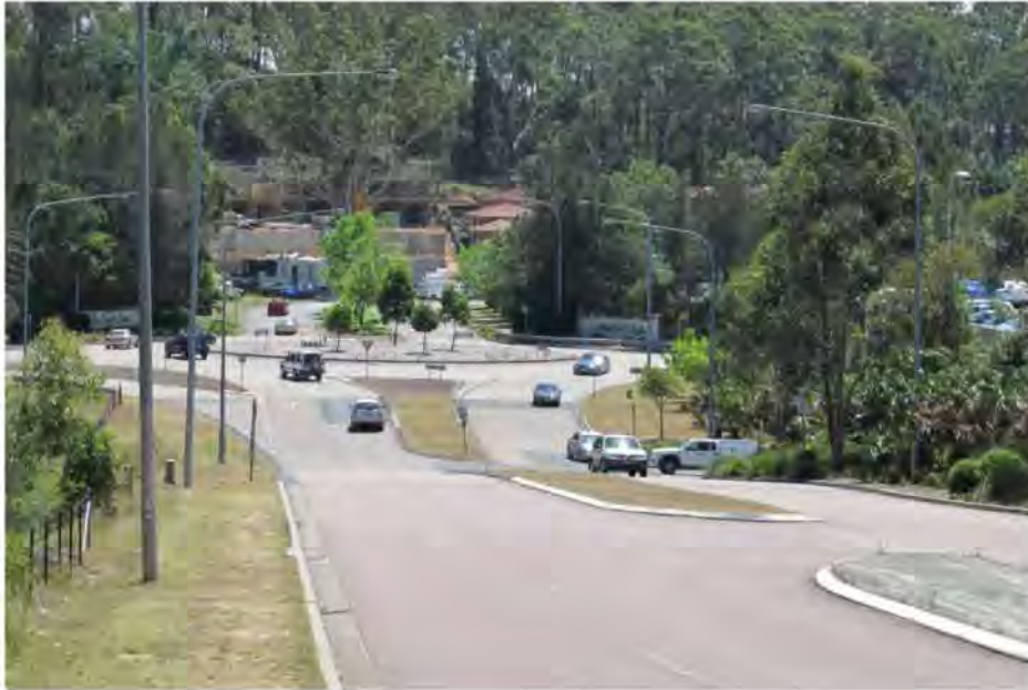
Figure 8. Tonkiss Street leading to the intersection with Wyong Road.
