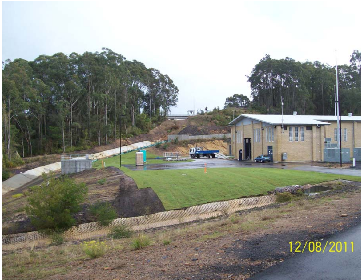
Restoration of the Mardi to Mangrove pump station site. (Work Package 6)
