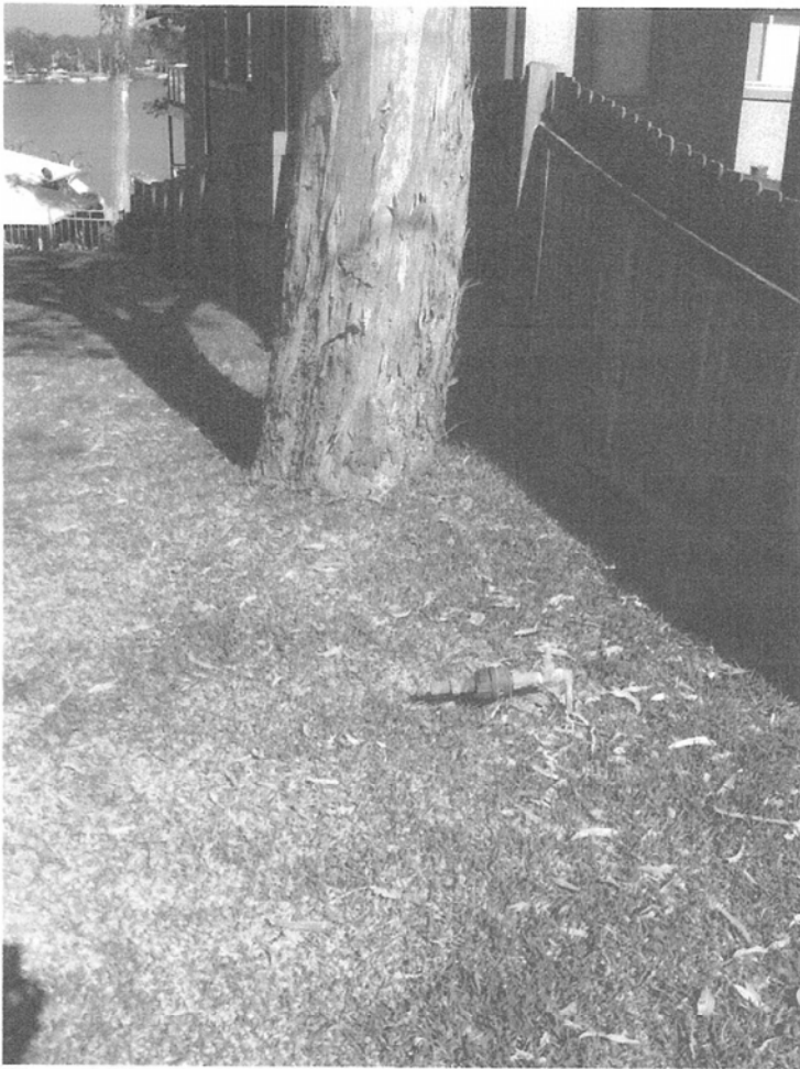
Photo.4 Showing location of the base of tree three. Note the location of water meter and the lean of the boundary fence.
