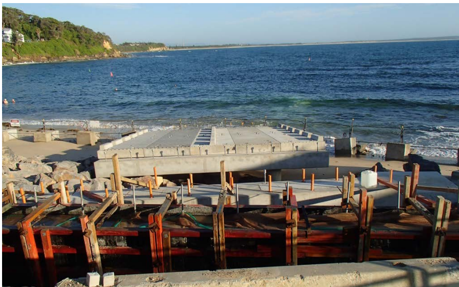
Construction of Norah Head boat ramp underway.
