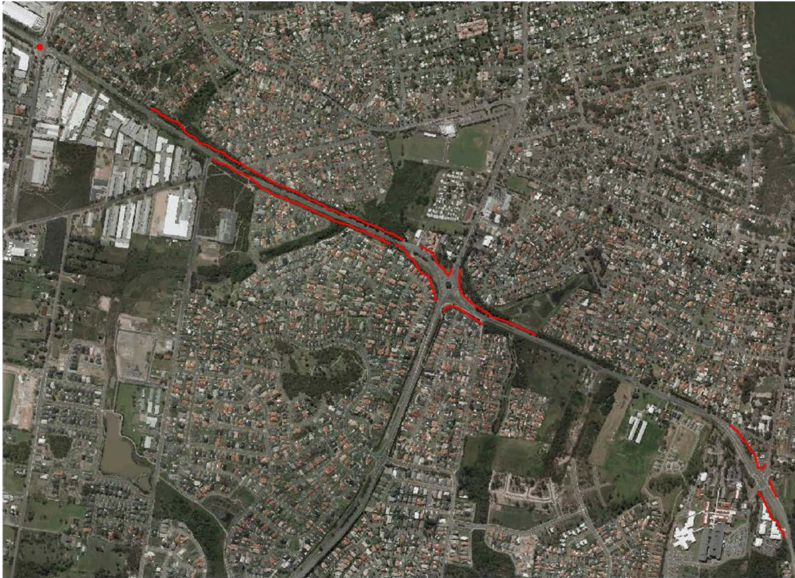
Pacific Hwy – Wyong Hospital to Lake Haven Roundabout
