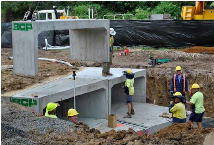
Wyong drainage works
