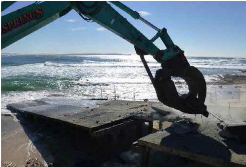
Norah Head boat ramp demolition
