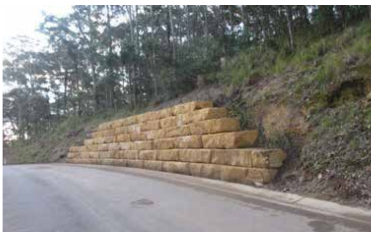
New retaining wall on The Ridgeway
