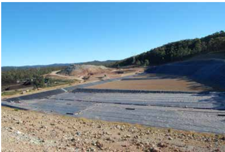
The new waste cell at Buttonderry Waste Management Facility
