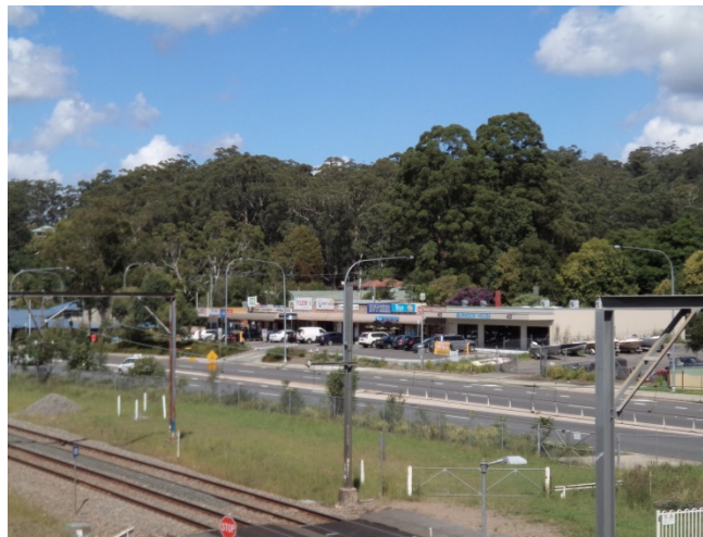
Figure 6: Looking south west from the railway footbridge to shops.
