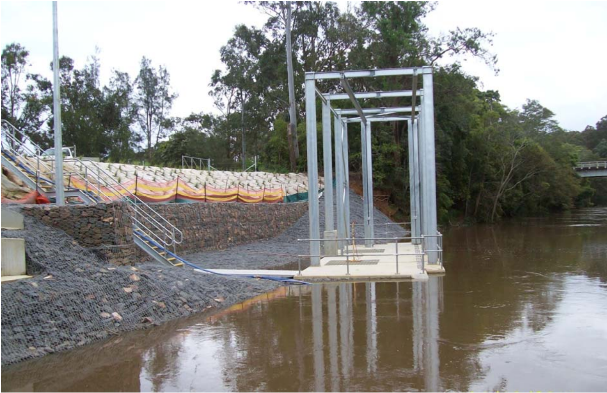
WP 01 Intake Tower (Work Package 1)
