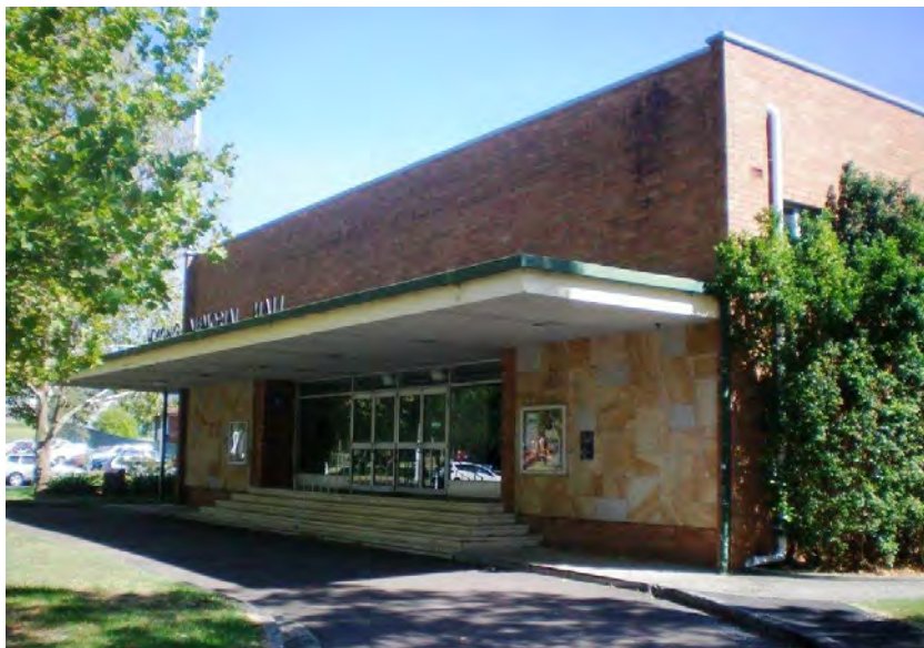
Existing memorial hall
