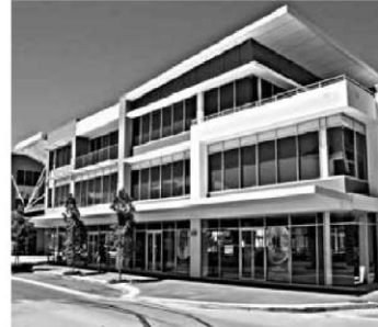
An example of low rise office building.
