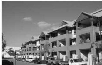
Built form that addresses the street.
