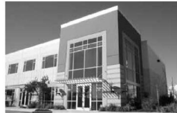
An example of low rise office building.
