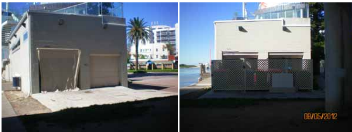
Figures 1 & 2: Site prior to and after the installation of screen fencing
