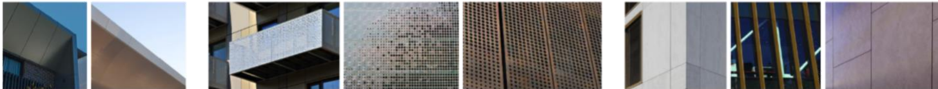
CLAD FACADES - Glazing slots - Aluminium panel cladding and louvre spandrels to window zones - Barestone or similar cladding panels
