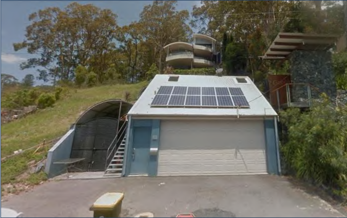
Figure 3 – Residential dwelling at 64 Araluen Drive
