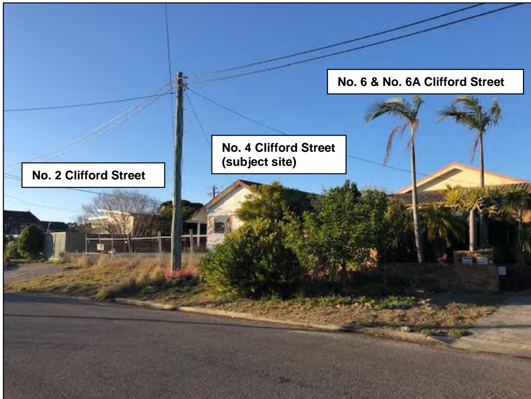
Figure 3 – Single storey residential dwellings adjoining the site
