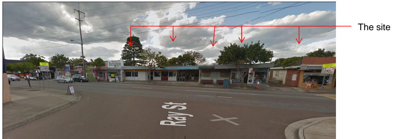
Figure 2 - Street view of Site
