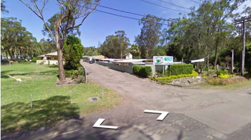
Child Care Centre - 433 Wards Hill Road EMPIRE BAY NSW 225
