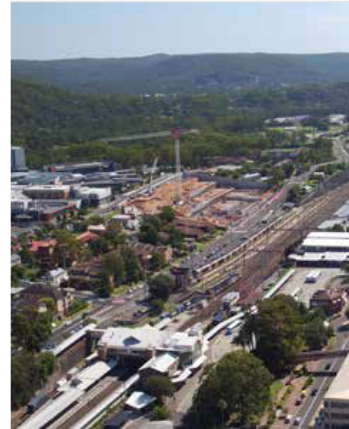
Gosford Hospital Precinct. Image: Bruce Downer
