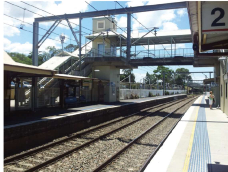
Wyong train station
