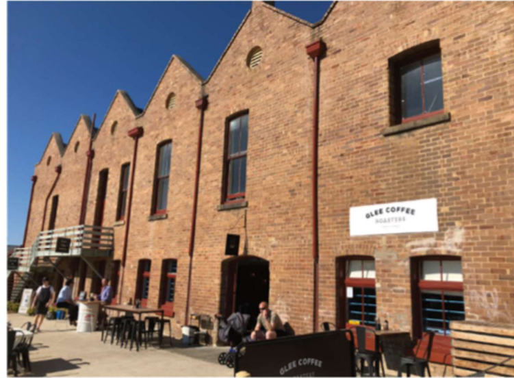
Chapman building, Wyong
