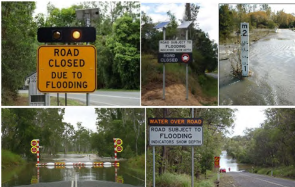
Image 23: Examples of Warning Signs, Boom Gates and Depth Indicators
