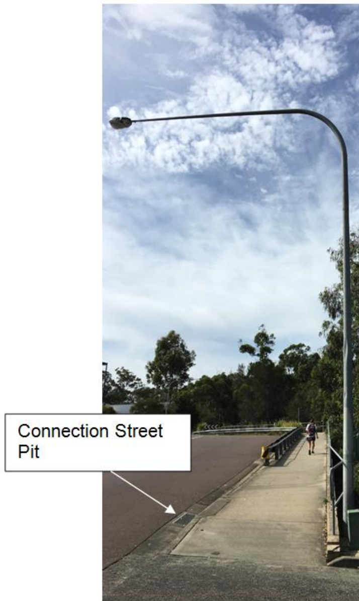
Figure 8 – Photograph of the downstream Stratford Avenue connection point.
