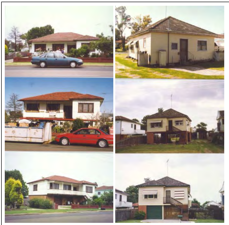
Plate 14 Examples of houses before (top image), during (middle image) and after (bottom image) house raising (photos courtesy of Fairfield City Council)
