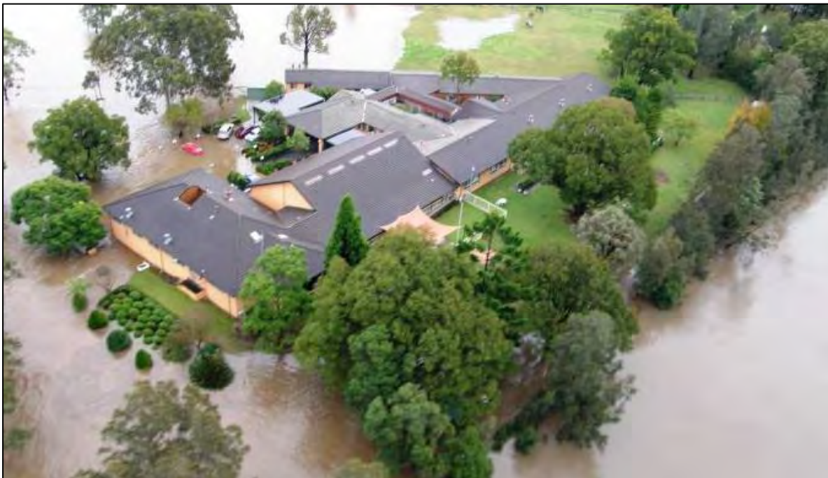
Plate 10 Wyong Aged Care Facility during 2007 flood showing all access roads inundated
