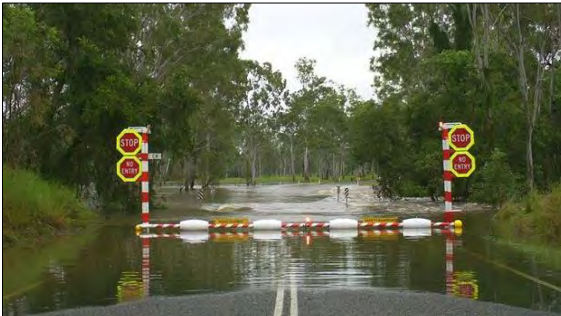
Plate 19 Examples of automatic flood barrier system (photo courtesy of David Bagnall)
